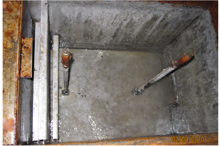
Interceptor pumped out - cleaned to standards.
